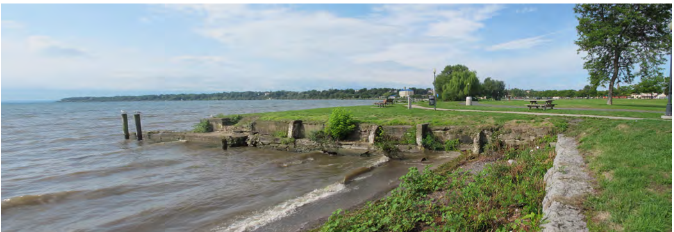
Figure 49: Existing beach location view
