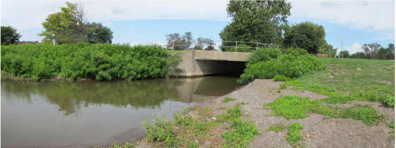
Figure 46: Existing Castle Creek outlet
