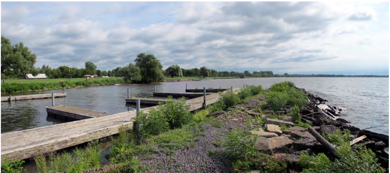
Figure 56: Existing Boat Launch breakwater
