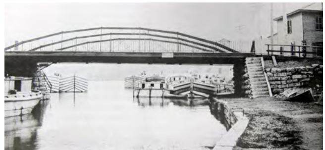
Figure 6: Whipple bridge over the Cayuga Seneca Canal
