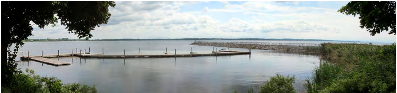
Figure 33: Existing Marina and Long Pier
