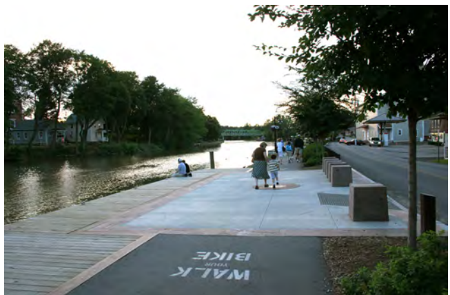
Figure 17: Integrated boardwalk and multiuse path along Pittsford Canal in Pittsford, NY
