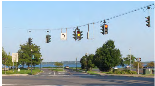
Figure 41: Existing Castle Street road alignment
