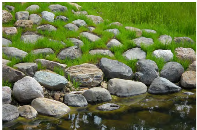
Figure 54: Photograph of proposed rip rap edging
